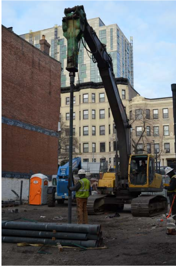
Figure 1. Picture of Ductile Iron Pile Installation
