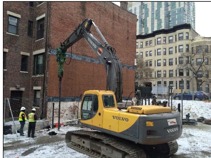
**Fig. 2. Ductile Iron Pile Installation**
