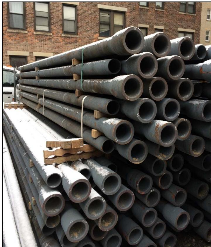
**Fig. 3. Ductile Iron Pile Material Stacked On-site**
