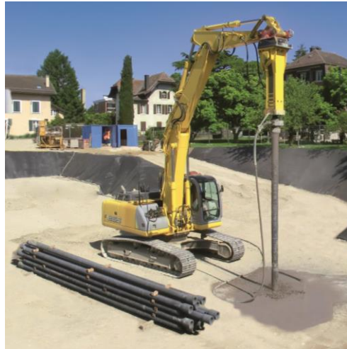
Figure 1: Ductile Iron Pile System
