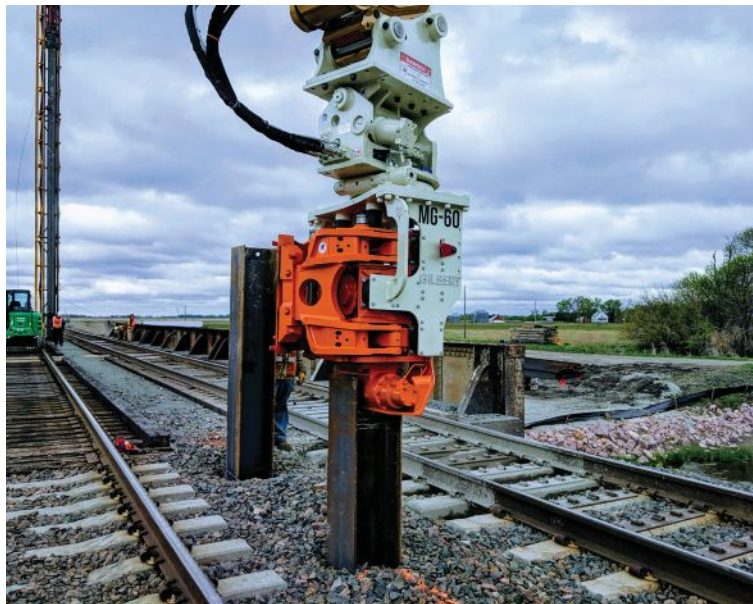
WORKING BETWEEN TWO RAILWAYS WITHOUT STOPPING TRAIN TRAFFIC Columbus, NE
