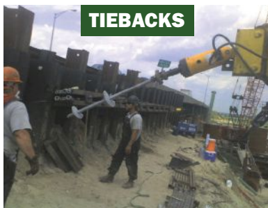
STELCOR DRILLED-IN DISPLACEMENT MICROPILES
