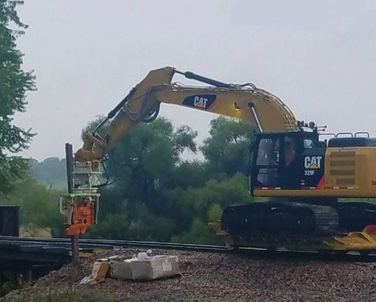
RAILWAY BRIDGE MAINTENANCE Des Moines, IA
