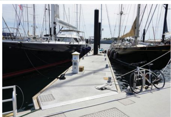
8' x 80' single cast concrete (one piece) finger w/ custom connection angle.
