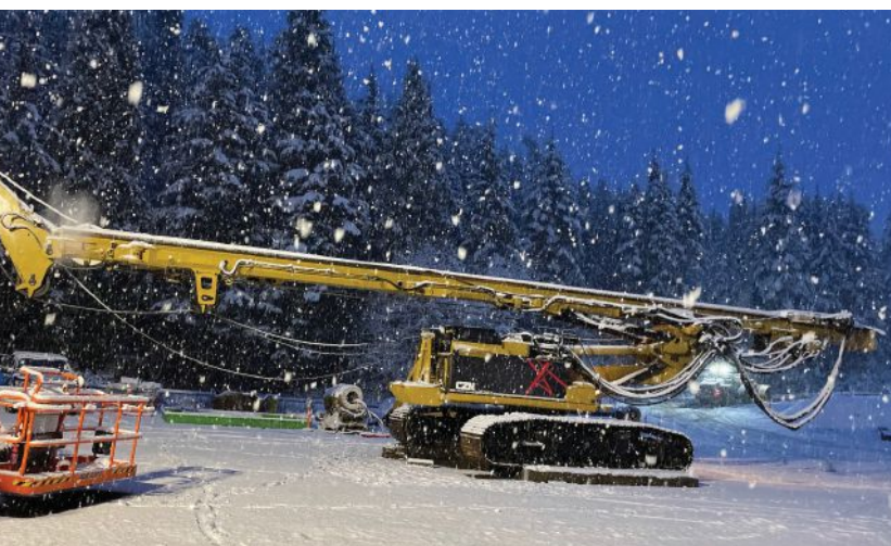
Drilling 200 ft depth in Kitimat, BC, Canada
