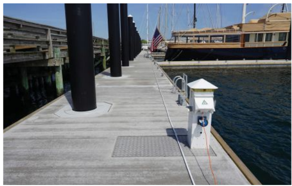
14' x 385' Floating Breakwater w/ off-center pile guides, and "Safety Pile Guide Cover."
