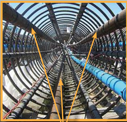
Also as Hollow Rebars for CSL Testing in Drilled Shafts "Patented"
