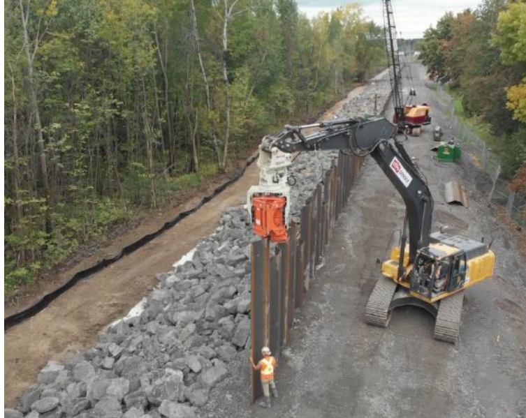
NEW DIKE REHABILITATION Quebec, CA
