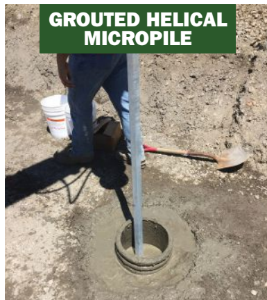
STELCOR DRILLED-IN DISPLACEMENT MICROPILES
