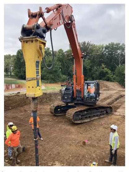
install the piles at an average rate of over 800 linear feet per day. Pile load testing on the job confirmed acceptable performance, providing the project team with a well-executed and successful value engineering deep foundation solution.
