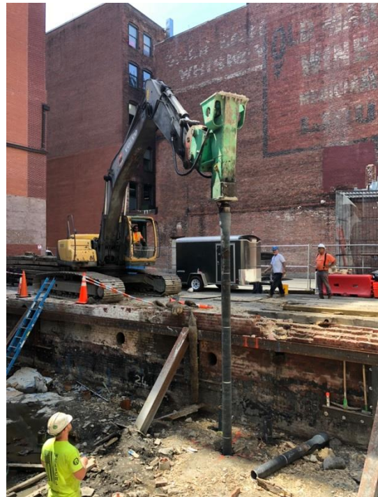
Figure 1: Ductile Iron Pile Installation
