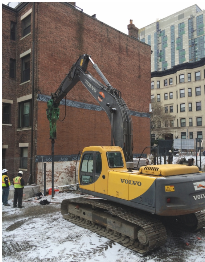
Pile installation near Fenway Park
