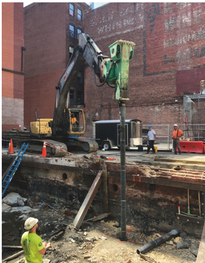
Pile installation near TD Garden
