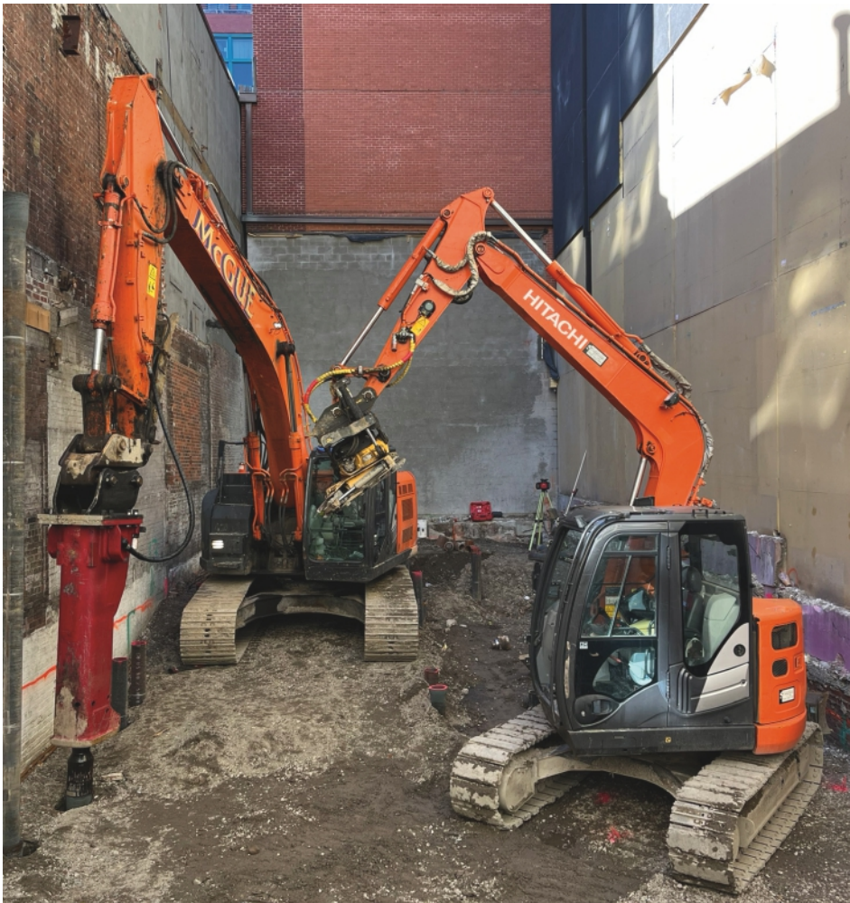
Pile installation near TD Garden
